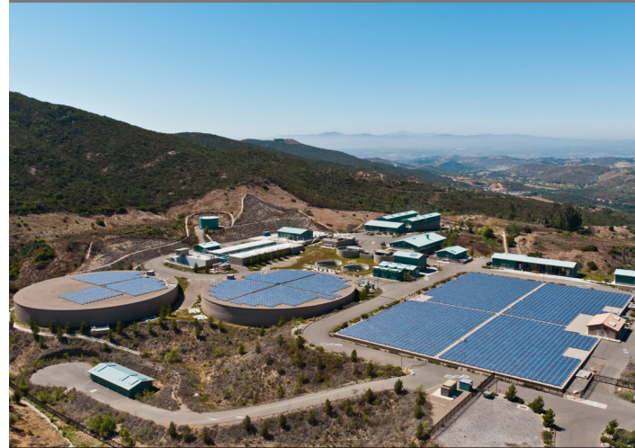
Solar panels at Twin Oaks Valley WTP
