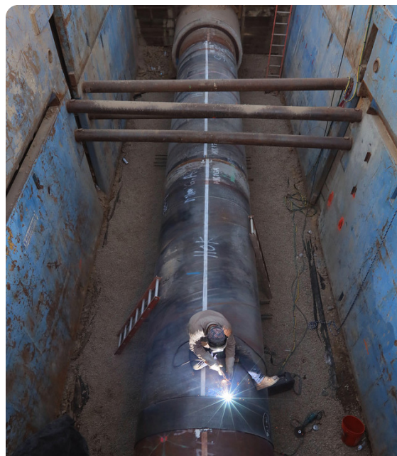
Typical Construction Project - Pipeline Rehabilitation with Steel Liners
