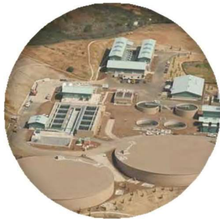
Twin Oaks Valley Water Treatment Plant
