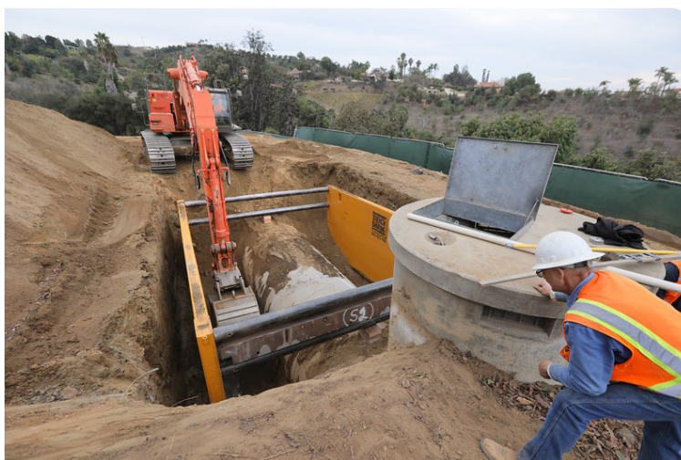
Typical Construction Project- Excavation and Backfill
