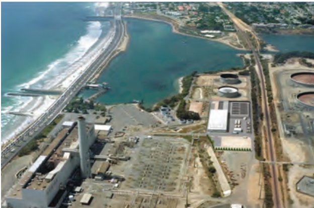
The Claude “Bud” Lewis Carlsbad Desalination Plant began commercial operation in December 2015, providing a highly reliable local water supply of up to 56,000 AF/year for the region.
