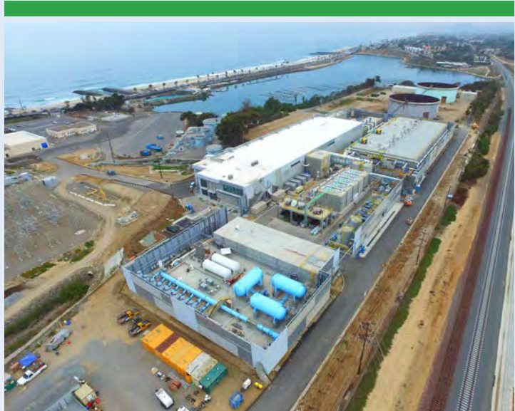
The Claude "Bud" Lewis Carlsbad Desalination Plant came on-line in December 2015. The Plant provides the San Diego region with a drought-resilient supply of water.
