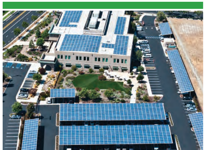
Solar panels at the Water Authority’s Kearny Mesa Headquarters produce renewable energy.
