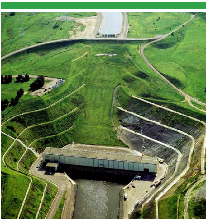
The Harvey O. Banks Pumping Plant pumps water south through the State Water Project to 25 million Californians.
