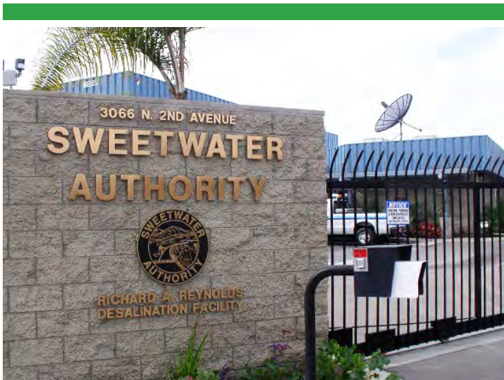
The Sweetwater Authority's Richard A. Reynolds Groundwater Desalination Facility is currently undergoing an expansion that will increase its capacity to 8,800 acre-feet per year.
