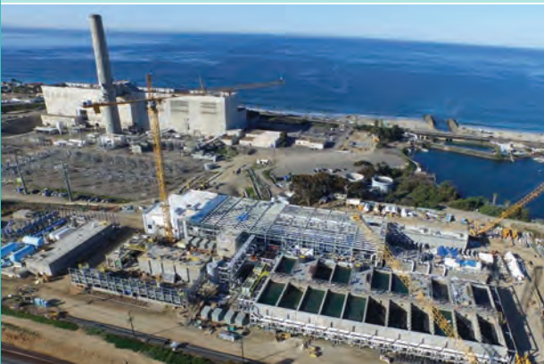
Claude "Bud" Lewis Carlsbad Desalination Plant under construction
