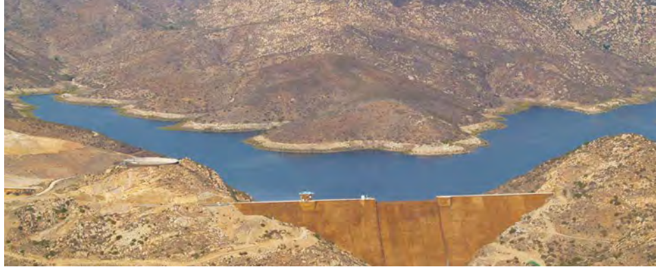
The San Vicente Reservoir Source Water Protection Project, sponsored by the Water Authority with funding from the San Diego IRWM Program, helps to maintain water quality in the expanded San Vicente Reservoir.
