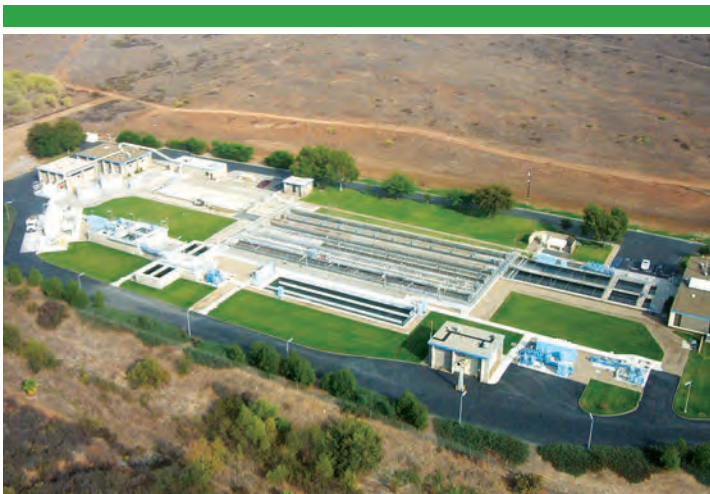
Padre Dam Municipal Water District’s Water Recycling Facility was upgraded in 1997 to treat two million gallons of wastewater per day.
