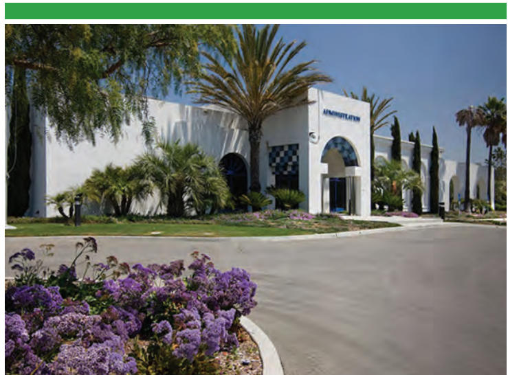
The City of Oceanside is expanding their recycling water system with a tertiary treatment capacity expansion of 0.8 MGD at the San Luis Rey Water Reclamation Facility.
