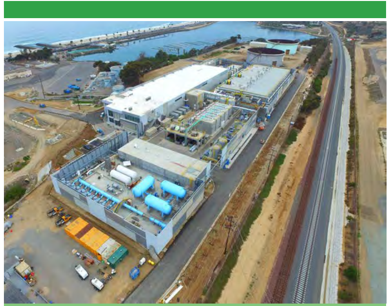
The Claude "Bud" Lewis Carlsbad Desalination Plant was certified by the SWRCB as a drought-resilient water supply for the San Diego region.
