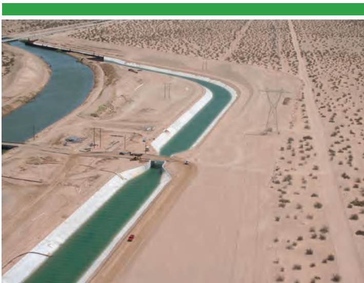
As part of the Quantification Settlement Agreement, the All-American Canal lining project began in 2005 and was completed in 2010.
