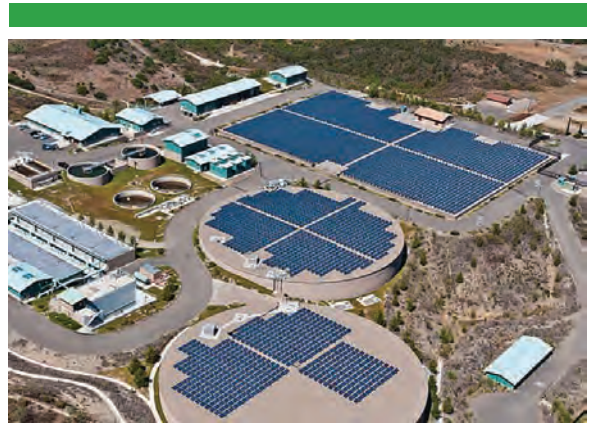
Twin Oaks Valley Treatment Plant
