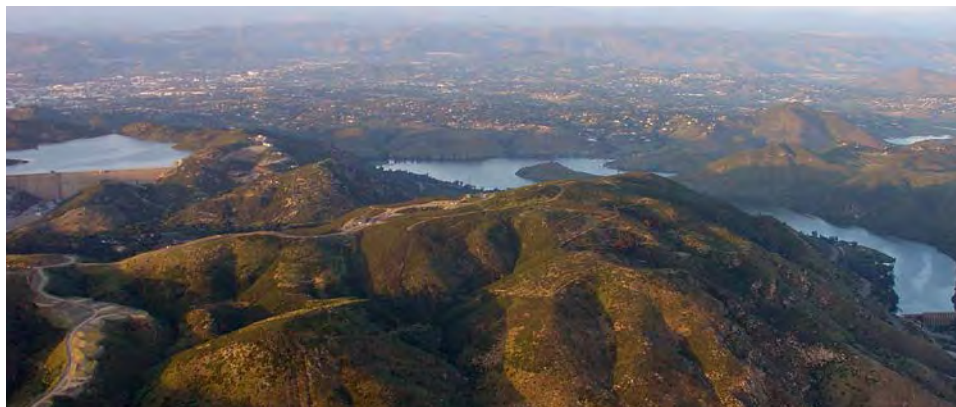
The San Diego IRWM Program is funding multiple projects that aim to solve water quality problems in the Hodges Reservoir.
