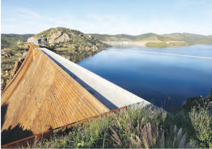
The carryover storage investment includes both surface water storage in San Vicente Reservoir and out-of-region groundwater storage in California's central valley.
