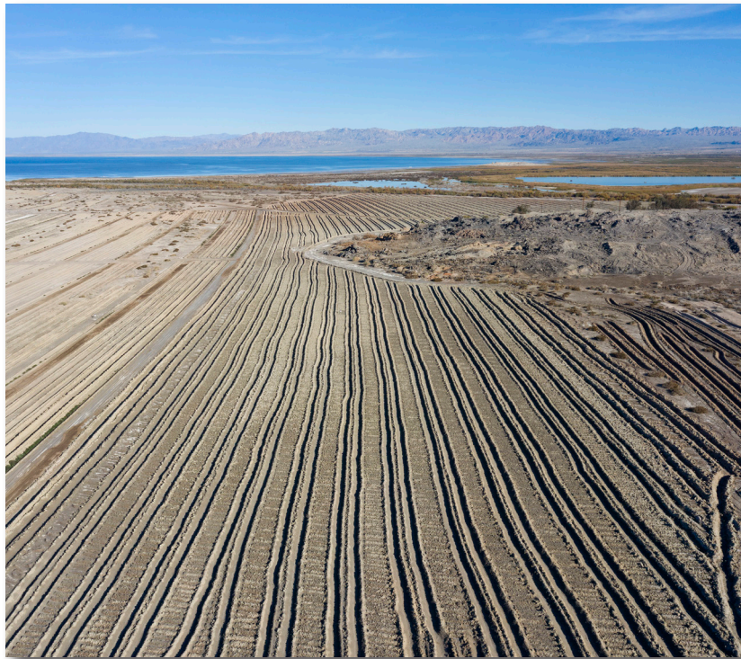
More than 1,300 acres of on-the-ground air quality projects, like surface roughening (pictured above) and vegetation enhancement, were completed in 2018. Another 1,000 acres is being established in 2019.
