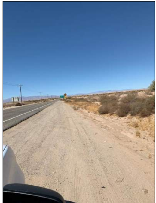
PHOTO 16: MP 8.4 looking west to north of SR78 near intersection of SR86.
