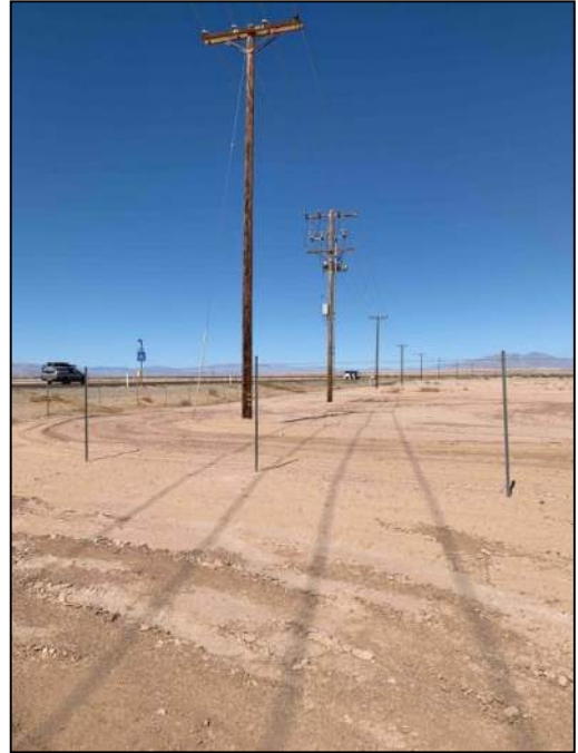
PHOTO 14: MP 6.8 looking north, east of SR86.
