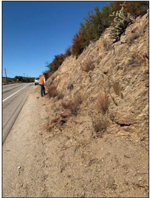
PHOTO 148: Cut into highly weathered metamorphic rock.
