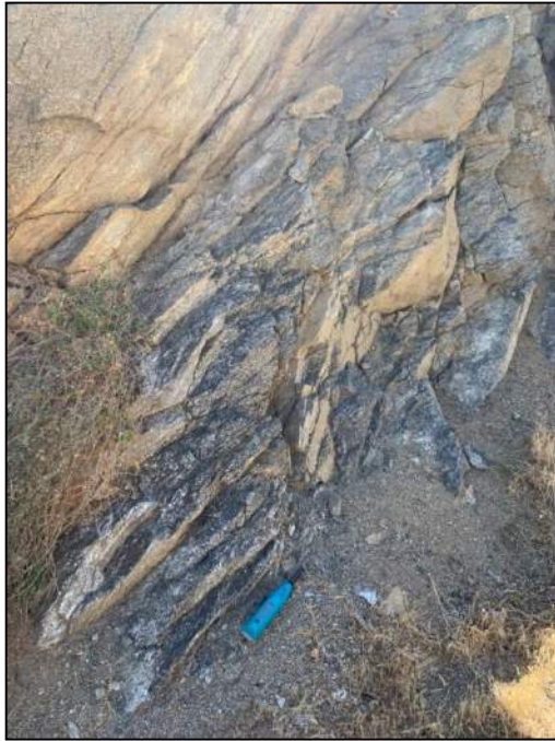
PHOTO 103: Closeup of cut in photo 101.
