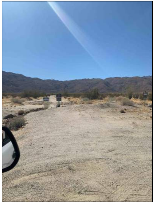
PHOTO 54: MP 40.2. View west approximately 0.5 Miles north of alignment down private road near S3. View is toward proposed tunnel portal in hillside.
