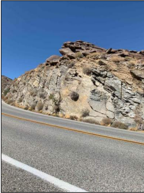
PHOTO 101: Cut in granitic rock with east dipping Foliation.
