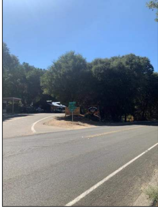
PHOTO 186: Near Lake Henshaw, looking west at Intersection of SR76 and Center Loop Road.
