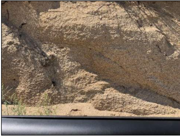
PHOTO 161: Cut into decomposed granitic rock.
