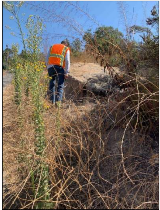
PHOTO 202: : Highly weathered granitic rock near MP 78.8.
