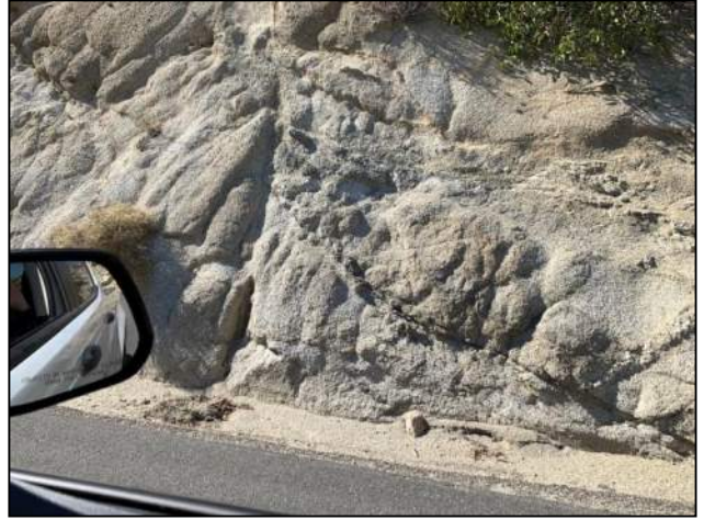
PHOTO 128: Cut in moderately to highly weathered granitic rock.
