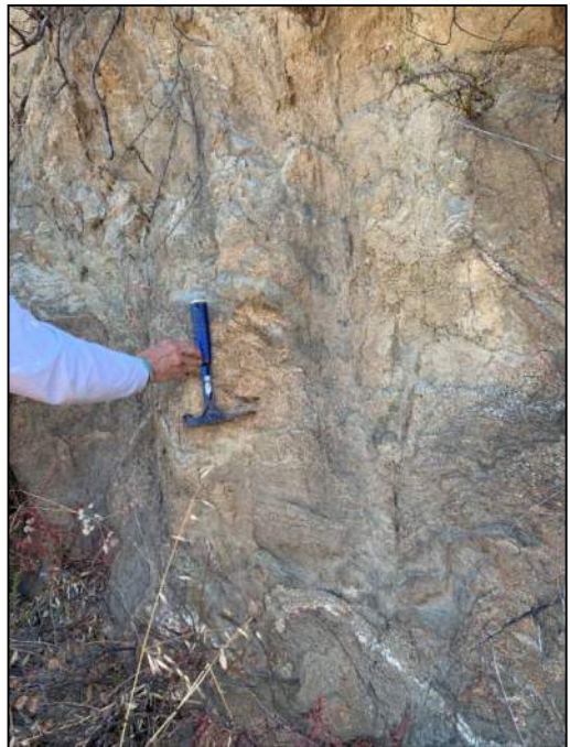
PHOTO 196: Highly weathered granitic rock in Cut on SR76.
