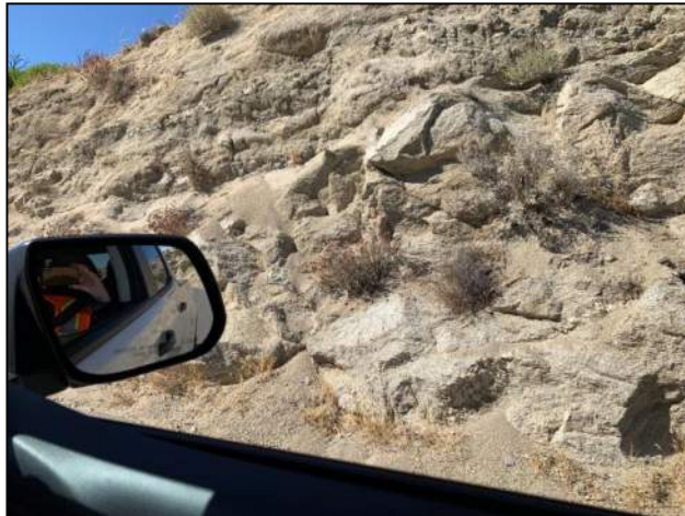
PHOTO 131: Cut in moderately to highly weathered granitic rock.
