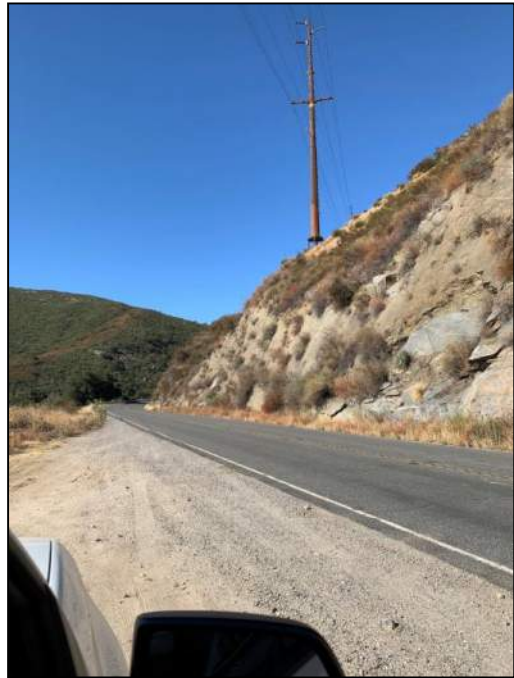
PHOTO 192: Cut of granitic rock west of Lake Henshaw.
