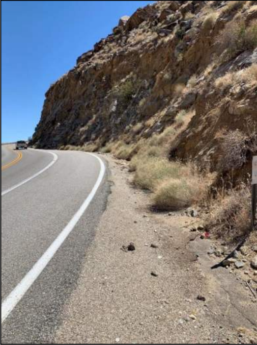
PHOTO 89: Steep cut in granitic rock.
