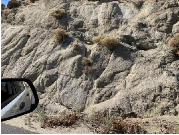
PHOTO 129: Cut in moderately to highly weathered granitic rock.
