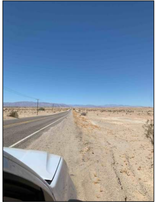
PHOTO 22: MP 9.7. View west of Roadcut.
