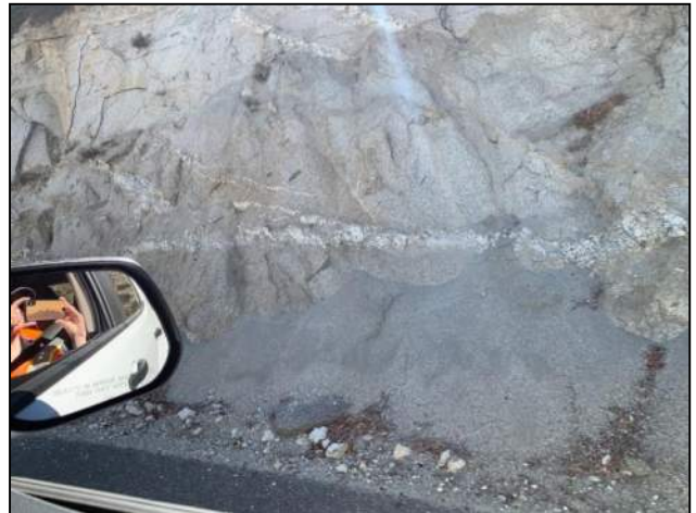
PHOTO 124: Cut in moderately to highly weathered granitic rock.
