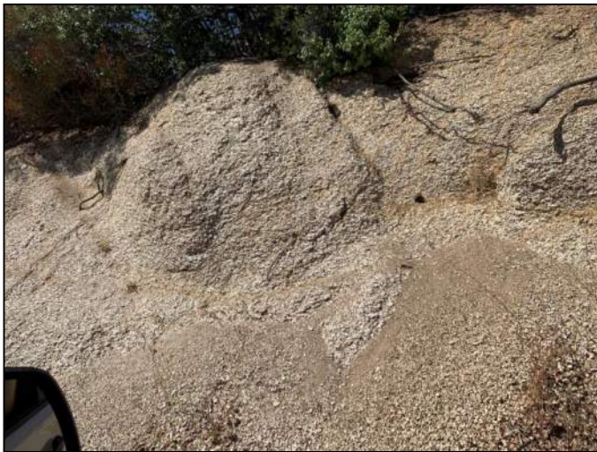
PHOTO 167: Cut into decomposed granitic rock.
