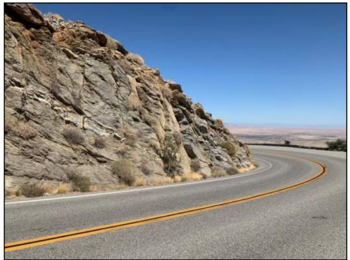
PHOTO 104: View looking east at desert overlook turnoff. This location is above the Tubbs Canyon Portal near MP 43.3.
