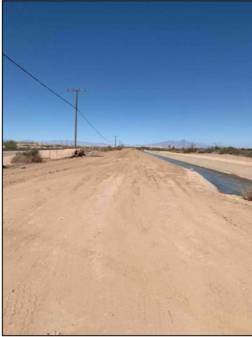
PHOTO 9: MP 3.6 looking north, east of SR86.
