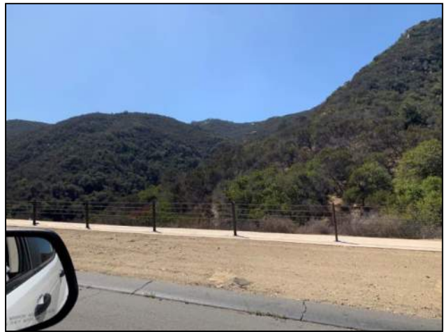
PHOTO 220: View looking west from I-15 just south of tunnel alignment.
