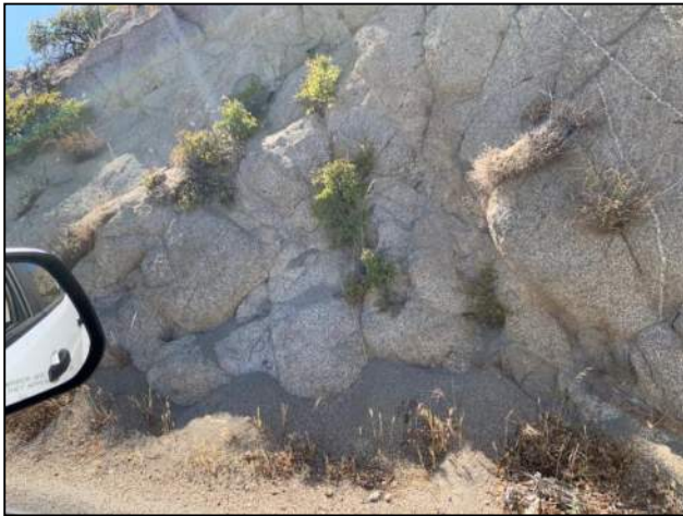
PHOTO 123: Cut in moderately to highly weathered granitic rock.
