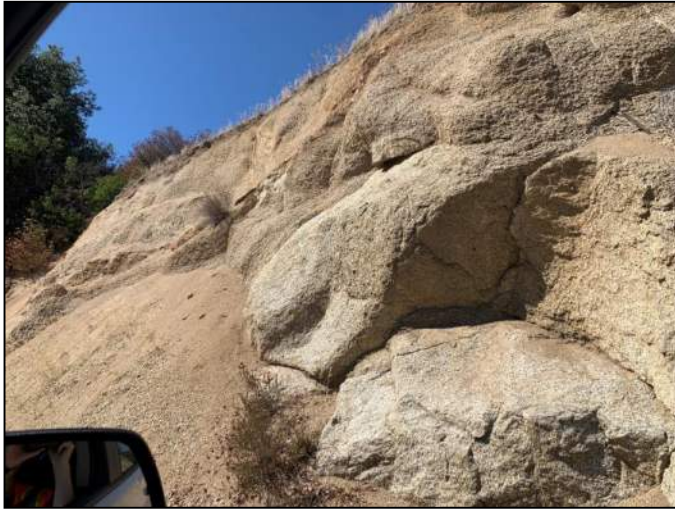
PHOTO 165: Cut into decomposed granitic rock.
