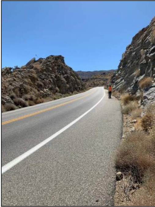
PHOTO 93: Slot cut in granitic rock.
