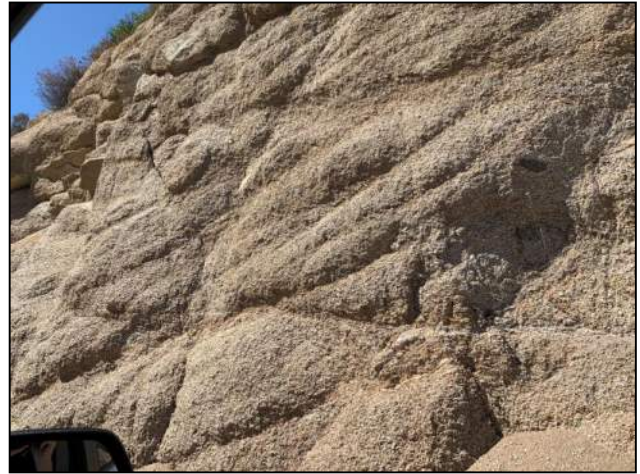
PHOTO 164: Cut into decomposed granitic rock.
