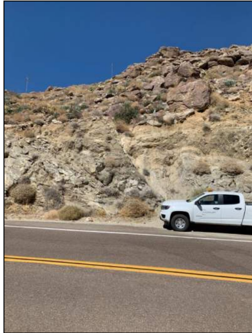
PHOTO 106: Possible fault in granitic rock. The front of the truck is at the locus of a steep east dipping fault structure. Notice the highly sheared rock material on the right side of photo.
