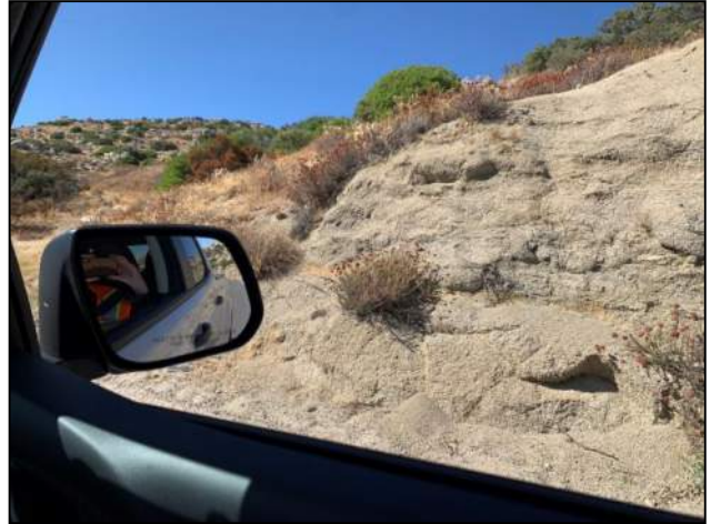
PHOTO 132: Cut in moderately to highly weathered granitic rock.
