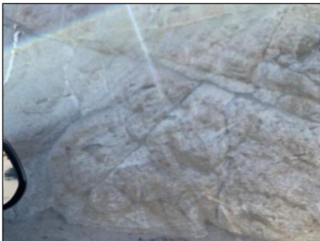
PHOTO 133: Cut in moderately to highly weathered granitic rock.
