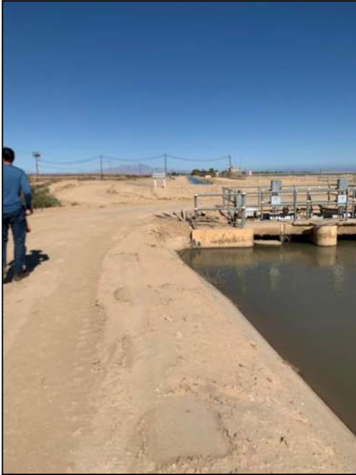
PHOTO 1. MP 0.0 Northern End West Side Canal (WSC).
