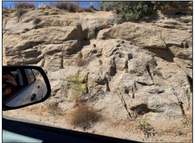
PHOTO 130: Cut in moderately to highly weathered granitic rock.
