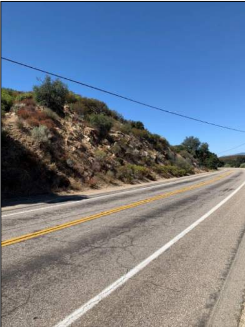
PHOTO 155: Cut containing both metamorphic and granitic rock.
