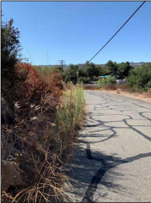
PHOTO 205: Area near tunnel alignment on Calle De Vista.
