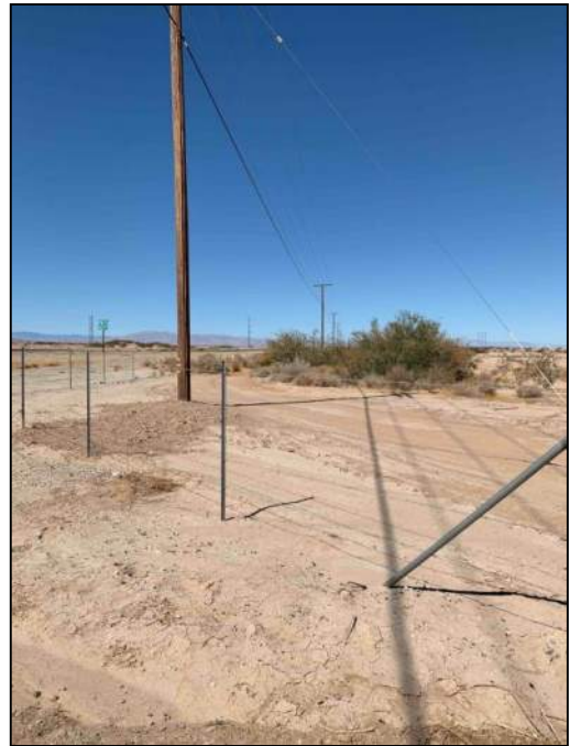
PHOTO 12: MP 5.7 looking north, east of SR86.
