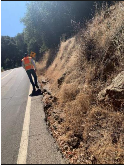
PHOTO 181: SR76 along south side of Lake Henshaw with road cut of granitic material.
