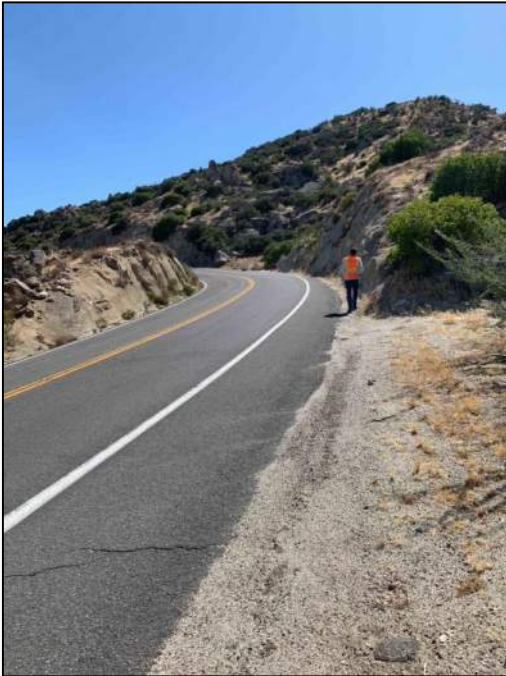
PHOTO 121: Cut of highly to moderately weathered granitic rock.
