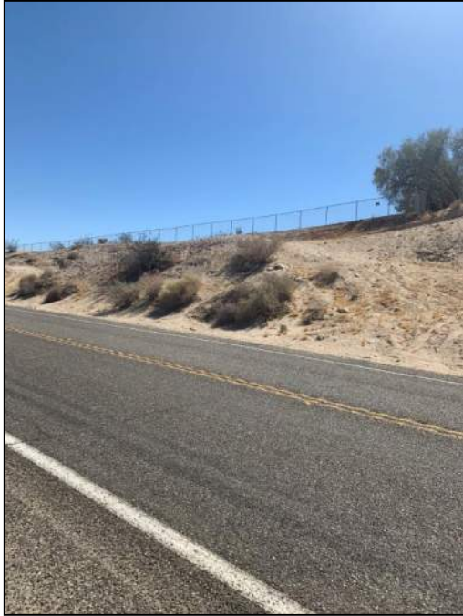
PHOTO 41: MP 24.5. View of roadcut on south side of SR78.
