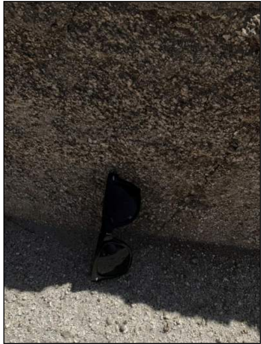
PHOTO 142: Decomposed granitic rock in cut on Lease Road.
