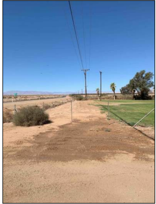
PHOTO 10: MP 4.6 looking north, east of SR86 at Elmore Ranch.
