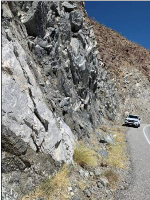
PHOTO 83: Steep cut in granitic rock. Notice weathered brown natural ground surface in background and fresh to slightly weathered gray rock in cut face.
