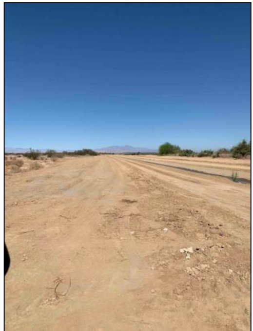
PHOTO 8: MP 2.5 looking north, east of SR86.
