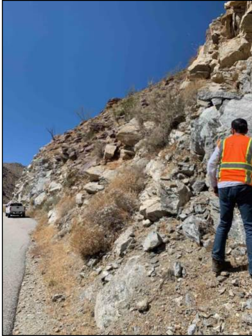
PHOTO 85: Cut in granitic rock.
