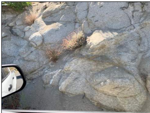
PHOTO 134: Cut in moderately to highly weathered granitic rock.
