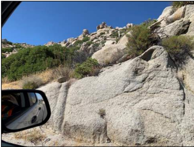
PHOTO 127: Cut in moderately to highly weathered granitic rock.
