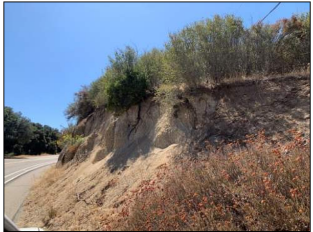
PHOTO 162: Cut into decomposed granitic rock.
