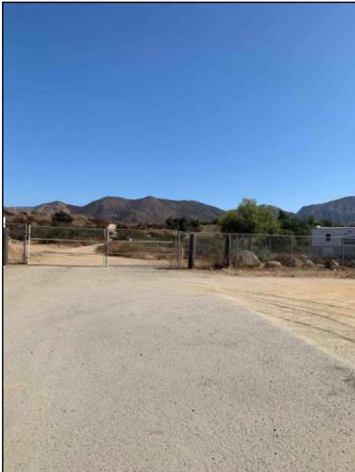
PHOTO 197: View looking east in area of tunnel alignment near North Lake Wohlford Road and Valley Center Drive.
