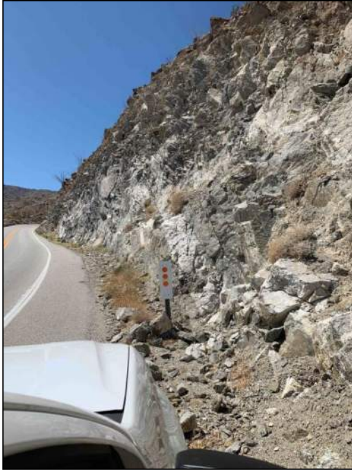
PHOTO 81: Highly fractured granitic rock.
