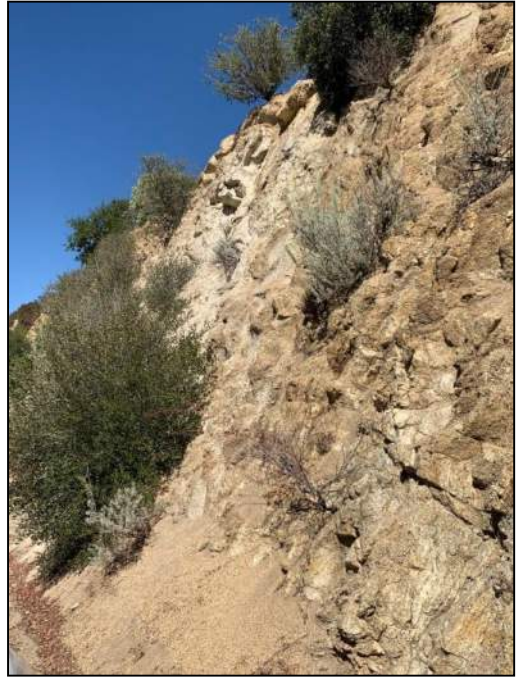
PHOTO 158: Same location as photo 157 looking West.
