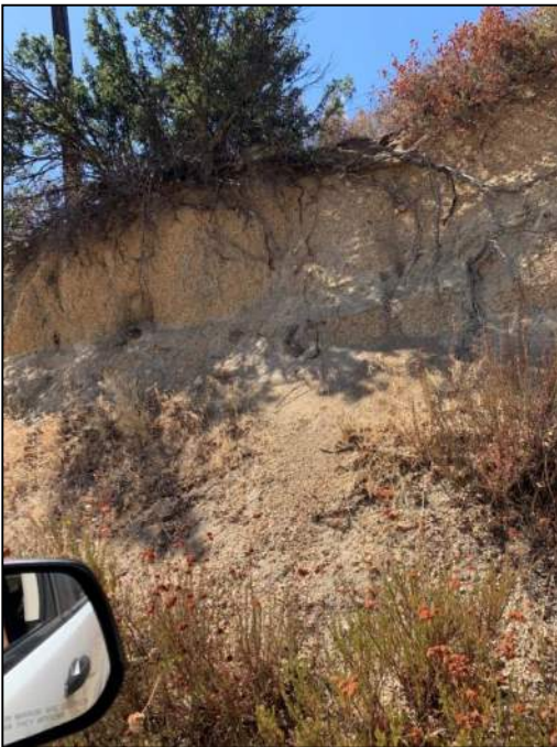
PHOTO 159: Cut into decomposed granitic rock.
