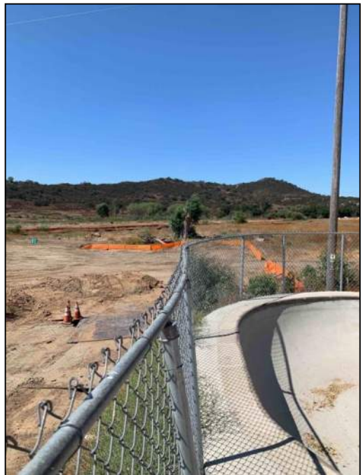
PHOTO 212: View looking west along tunnel alignment at Valley Center skate park.
