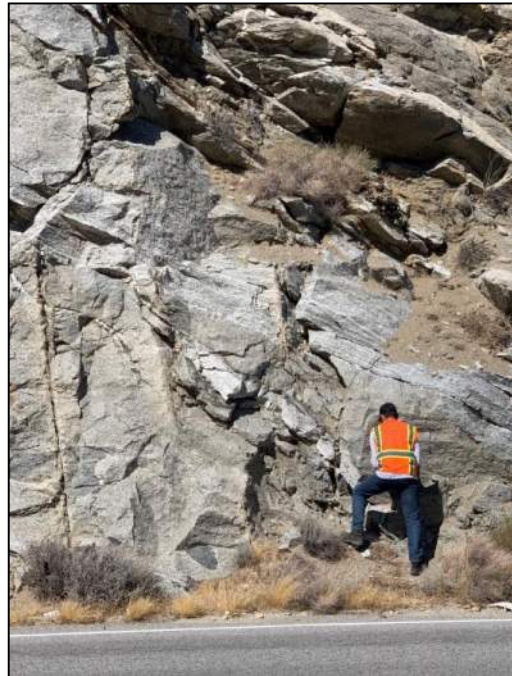
PHOTO 108: Close up of photo 107.
