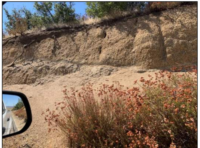
PHOTO 160: Cut into decomposed granitic rock.
