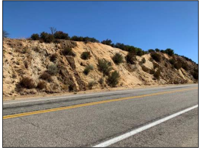
PHOTO 150: Cut on north side of S22 west of Ranchita. The cut is in a contact zone with both metamorphic and granitic rock.
