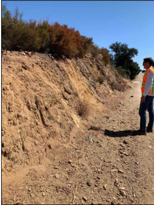
PHOTO 145: Cut in highly weathered metamorphic rock west of Ranchita on S22.
