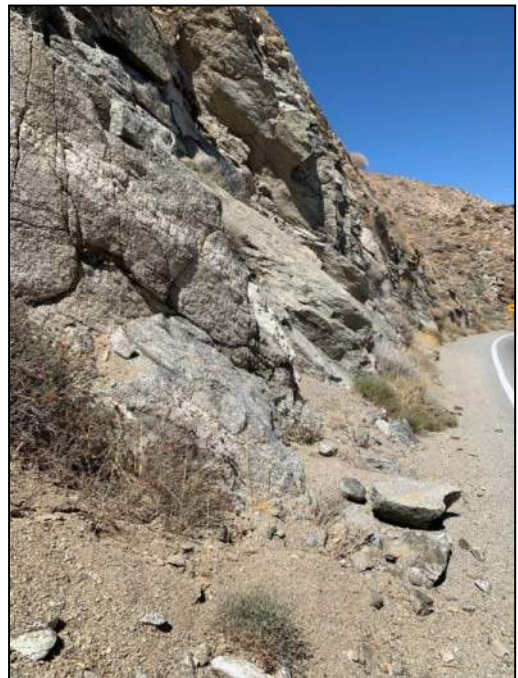
PHOTO 94: Cut in moderately weathered granitic rock.
