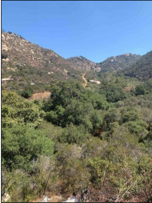
PHOTO 213: View looking east from Old Highway 395 along cut and cover section up to portal area at MP 79.3.
