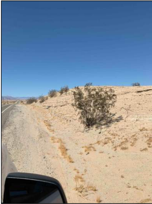
PHOTO 21: MP 9.7. Overview of Roadcut of Brawley Formation on north side of SR78.
