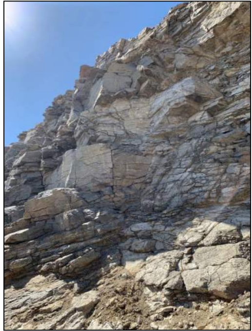
PHOTO 98: Closeup of cut in photo 97.
