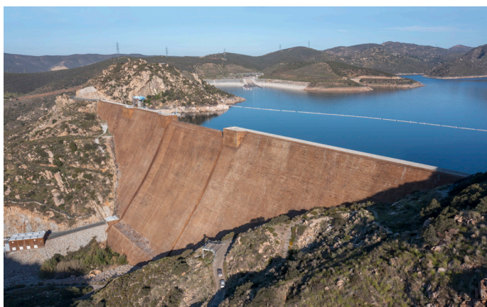
San Vicente Dam
