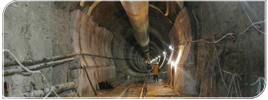
47 Miles of Tunnels
