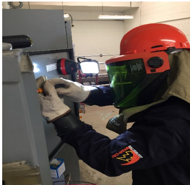
Figure 14 – Mission Trails Flow Regulatory Structure Electrical PM
