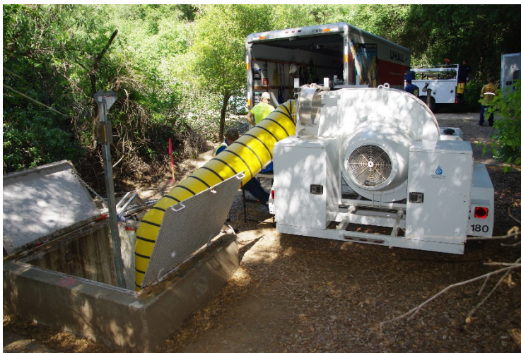
Figure 6 – 1 st Aqueduct Pipeline Condition Assessment
