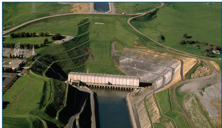
The Harvey O. Banks Pumping Plant pumps water south through the State Water Project to 27 million Californians.
