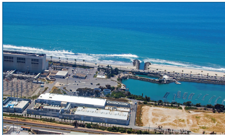
The Claude “Bud” Lewis Carlsbad Desalination Plant began commercial operation in December 2015, providing a highly reliable local water supply of up to 56,000 AFY for the region.
