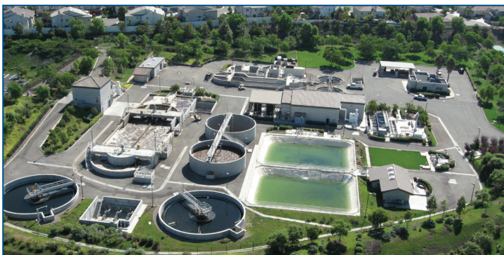
Water reclamation plants, such as 4S Ranch Water Reclamation Plant (shown), produce recycled water for non-potable irrigation and industrial uses. Photo credit: Olivenhain Municipal Water District
