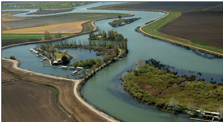
In the Bay-Delta, levees both provide flood control and act as channels to convey water to the pumps in the Southern Delta for export to Southern California and the San Joaquin Valley.
