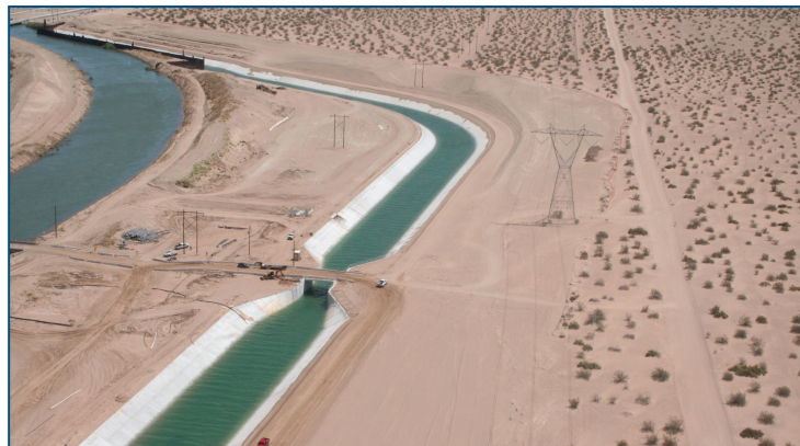
Concrete-lined portion of the AAC. Conserved water from lined portions of the AAC and CC provide the San Diego region with a drought-resilient supply.
